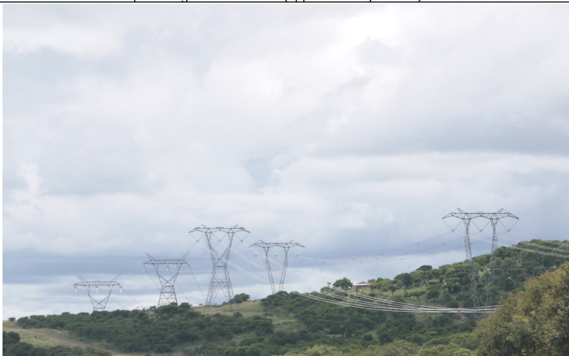
Plate 10 - Existing 400kV double overhead transmission lines are highly obvious as they cross ridgelines from short distance (approximately 1km).
