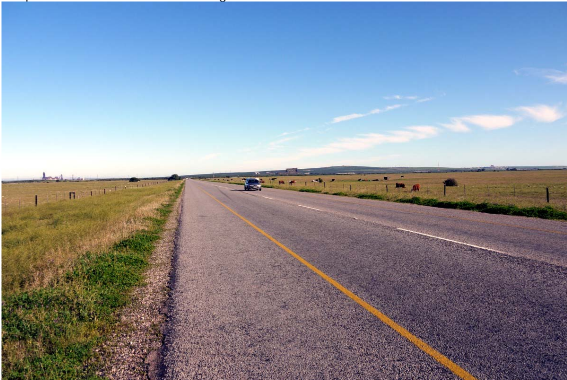
Plate 22, Viewpoint 9 - A view looking west along the local road that connects the R27 and R399. TX substation alternatives D and F will require 132kV power line running along the RHS of the road.
