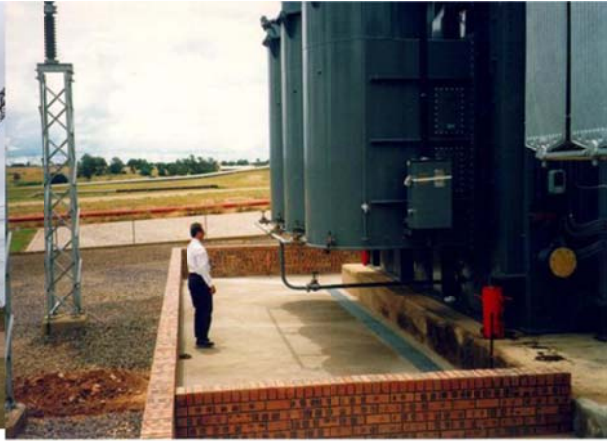
Plate 2 – Transformer approximate height 8m
