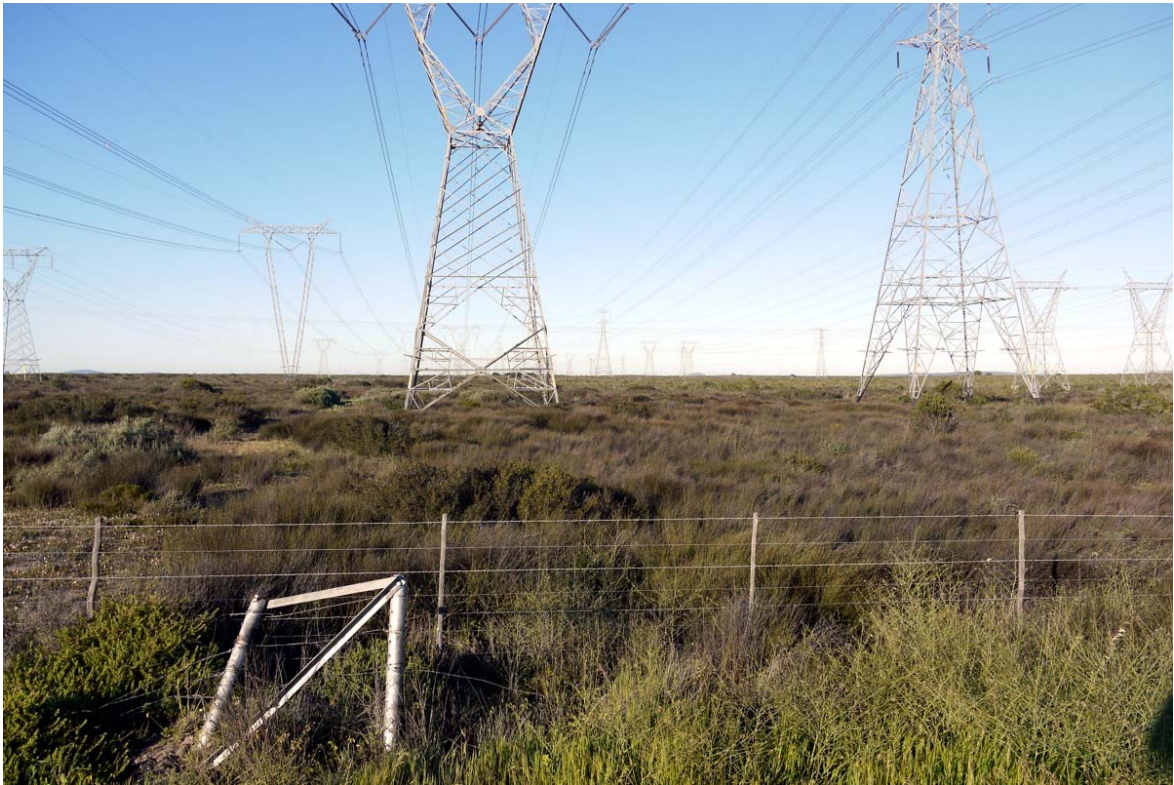
Plate 13, Viewpoint 1 - a view along the existing power line servitudes looking west from the Aurora Substation. The proposed 400kV overhead power line alternatives will run close to and parallel with these existing power lines.
