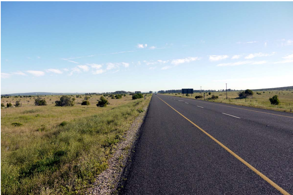
Plate 16, Viewpoint 4 - A view looking along the R27 from close to the point that alternative 400kV power line alternatives 4 and 6 join the road looking north. These alternative alignments will result in 400kV power lines running close to and parallel with the right hand side of the road.
