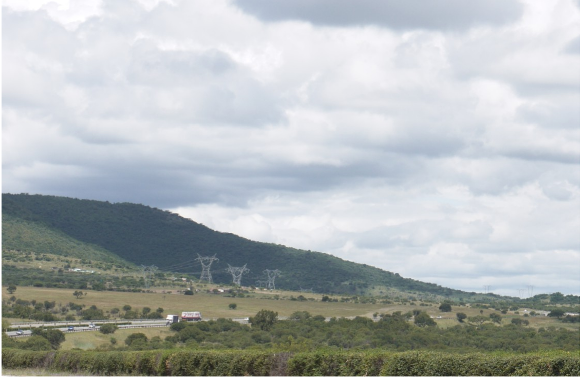
Plate 11 - Existing 400kV overhead transmission lines. Towers are obvious in the mid distance (approximately 2-3km) but are not highly conspicuous at a distance (approximately 5-6km) as they cross the ridgeline.
