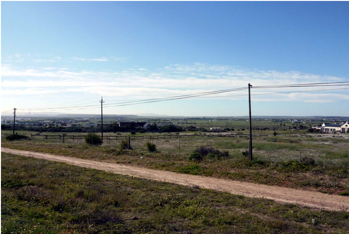
Plate 23, Viewpoint 10 - A view looking north from the Saldanha to Langebaan Road close to Mykonos towards the TX substation alternatives at a distance of approximately 4km. Note, existing 400kV overhead power lines are not obvious. Proposed infrastructure is also unlikely to be obvious from this viewpoint.
