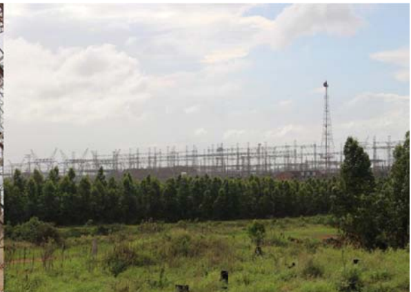
Plate 4 - Sub-station & Communication Tower
