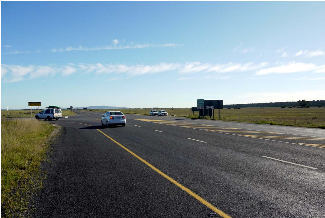
Plate 19, Viewpoint 7 - A view looking north along the R27 towards TX substation alternative sites D from a distance of approximately 400m. Alternative D will be seen just behind the two parked police cars centre image and approximately 40m from the road edge.
