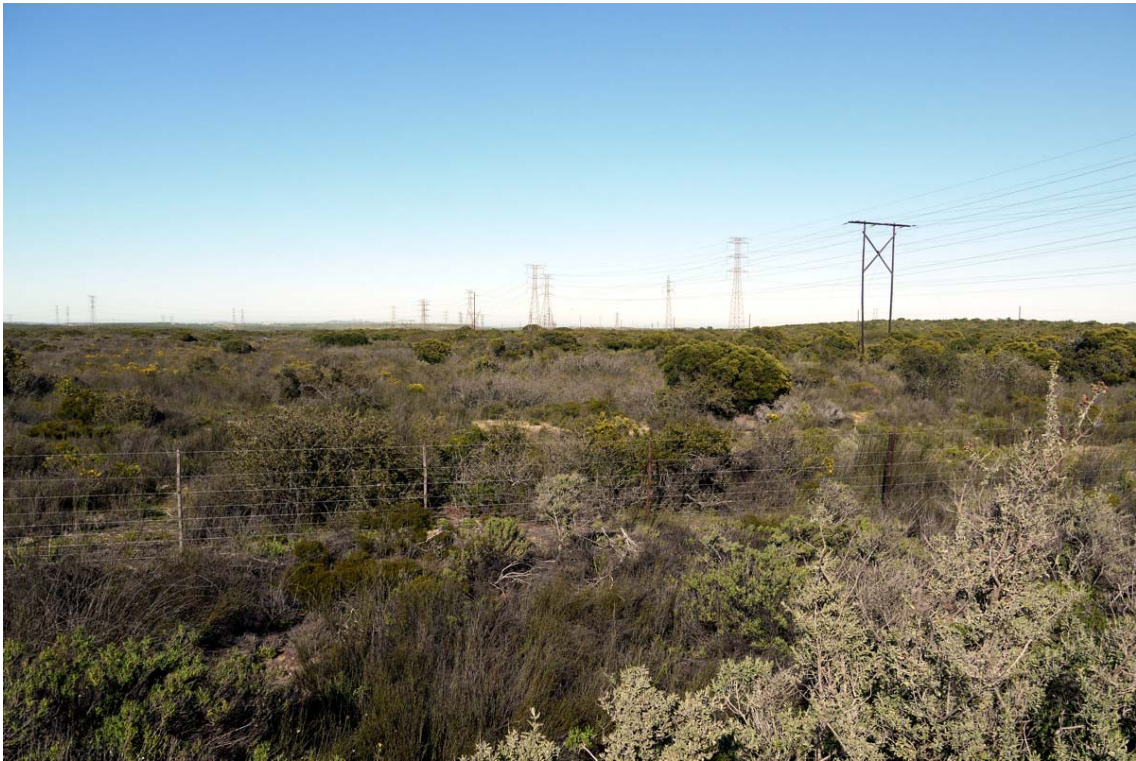
Plate 21, Viewpoint 8 - A view looking south from the local road that connects the R27 and R399 looking at the existing Blouwater DX Substation (centre image to RHS of two 400kV towers). The existing substation is largely screened by minor undulations in the landform. Alternative DX substation A will also be well screened from this viewpoint. Alternative B is also likely to be partially screened. Alternative C will be highly obvious from this road being located approximately 100m from the viewpoint and just to the left of centre of the image.
